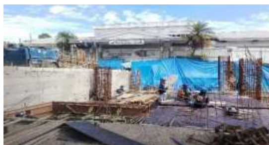
Gambar 6: Bekisting Pelat Lantai
