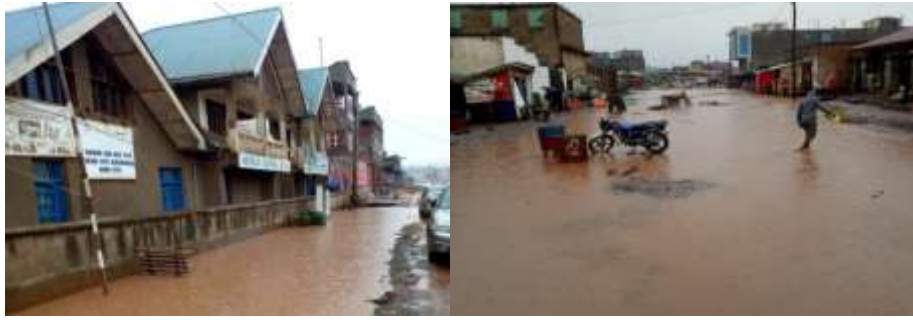
Figure 4. Overview of the state of the Butembo Health Zone office and the flooding of the squares occupied by the Makasi market.
