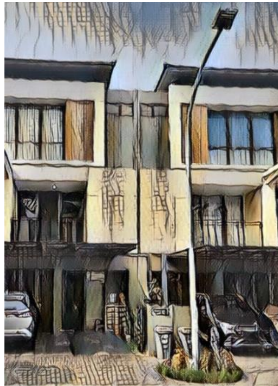
Figure 3. Street lights on The Zora Residence
