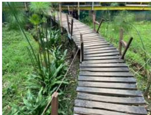
Figure 1. Bridge to Glamping area (Source: Personal)
